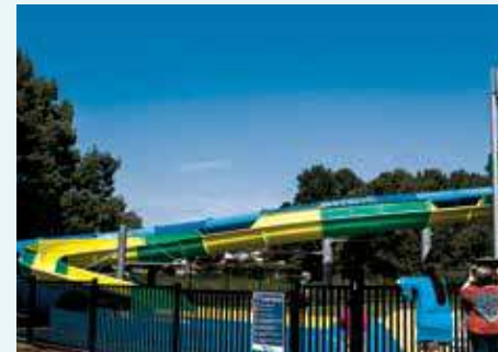
Nowra Aquatic Centre, NSW
